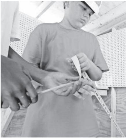
Hard hat-wearing D.J. Felton, one of about a dozen kids participating in the camp, straightens out a tape measure inside a garden shed under construction.
